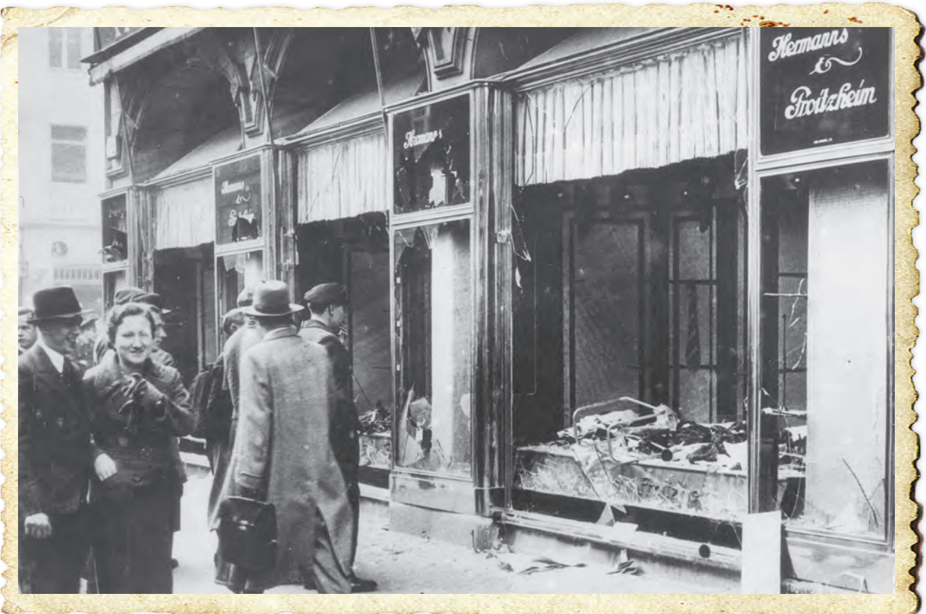
Wrecked and pillaged windows of Jewish shops in Friedrichstrasse, Berlin, after the November Pogrom 1938. Courtesy Wiener Library.
